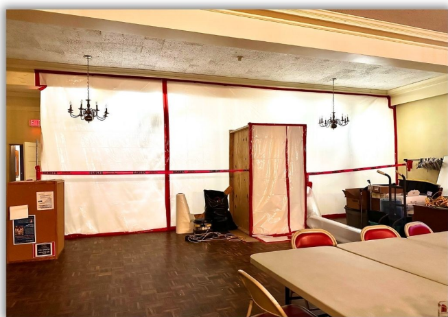
Asbestos abatement at the beginning of the project
