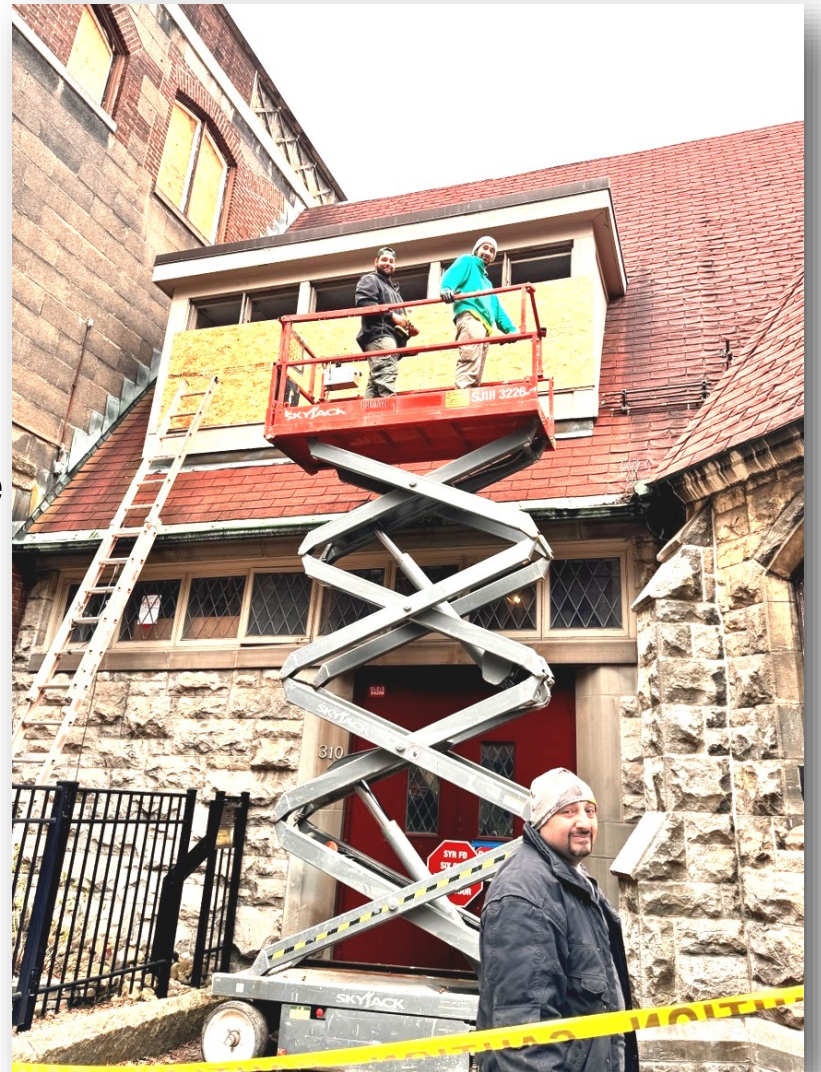
Parish House windows will be removed and restored
