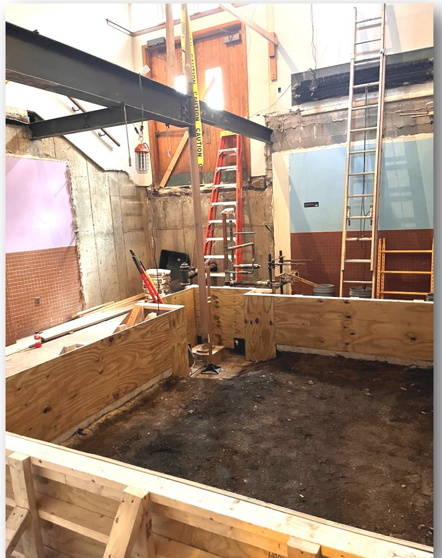
Preparing for the foundation for the elevator shaft.
