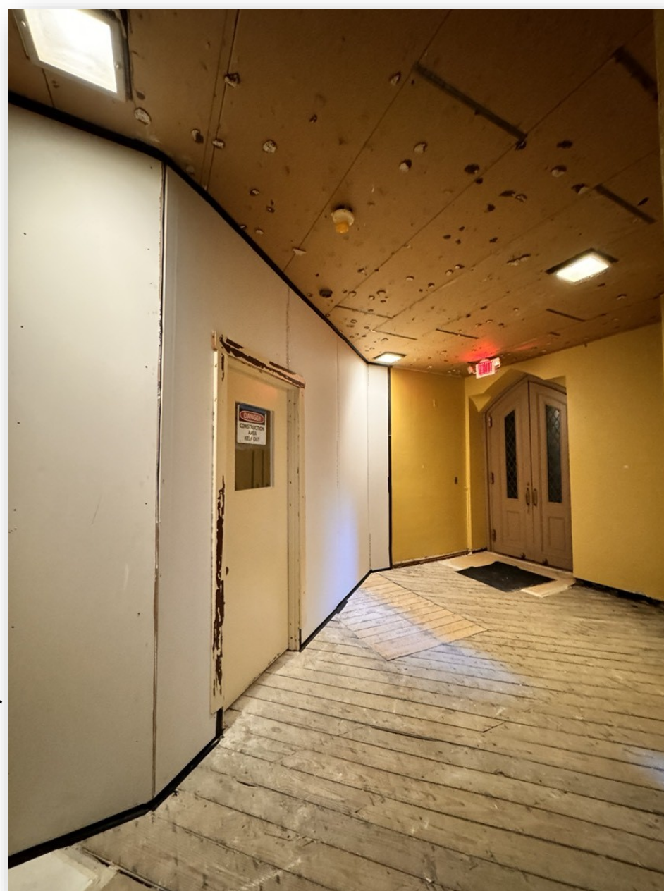
The Sargent Foyer is sporting a new temporary wall. This will protect the sanctuary from dust and such during the installation of the new exterior door.
